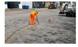
This allows the concrete to have contamination removed off the surface easily and remain looking like a clean concrete pad.
