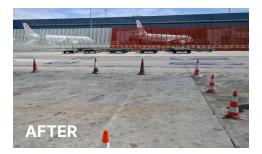
Spray-Lock SCP 743 was used over three successive applications to lift out the vast majority of this embedded contamination through its Calcium Silicate Hydrate (C-S-H) reaction within the concrete when applied into the concrete capillaries.
