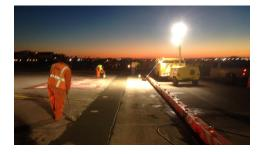
ShieldCrete® SCP-743 treated the rapid cure concrete at time of concrete placement. It was reported that significantly less cracking was observed when compared to other concrete strips laid in past concrete pours.
