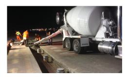
A Rapid cure concrete solution was required at the hold fast strip on the main runway at Los Angeles Airport (LAX). This concrete strip is 450 mm thick, and used with fast cure concrete. To provide a rapid cure of concrete solution and to also protect the concrete from all forms of attack.
